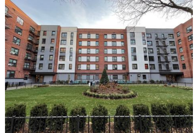
Site improvements at Warren St Houses
