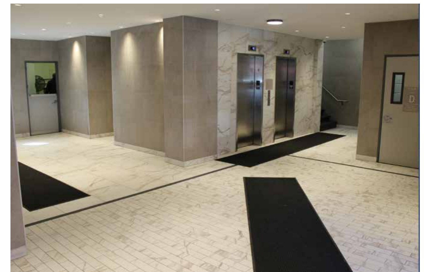
Renovated building entrance at Warren St Towers
