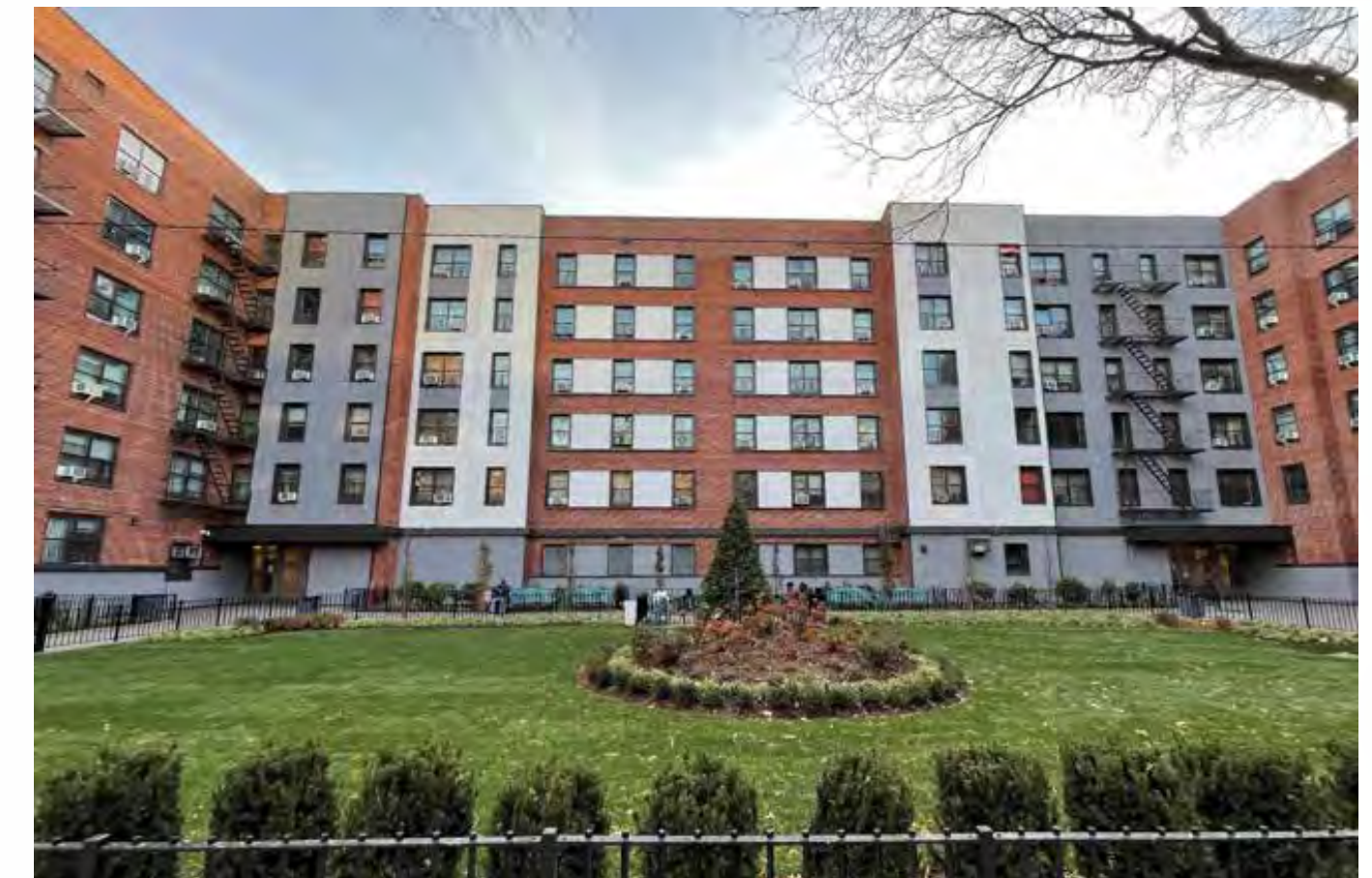
Site improvements at Warren St Houses
