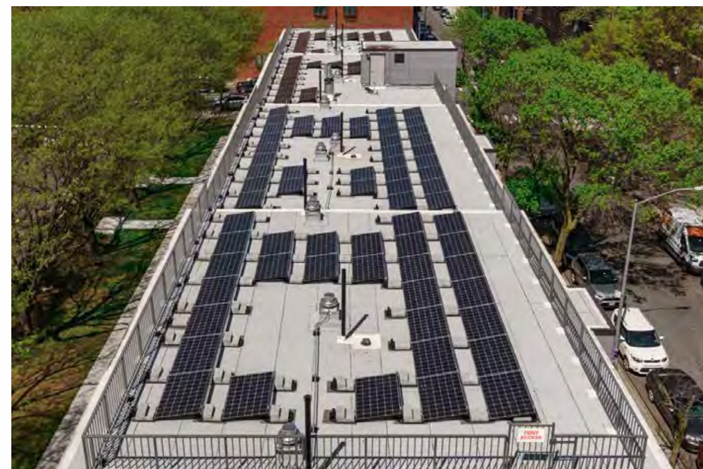
Repaired roof and solar panel system at Berry St Houses
