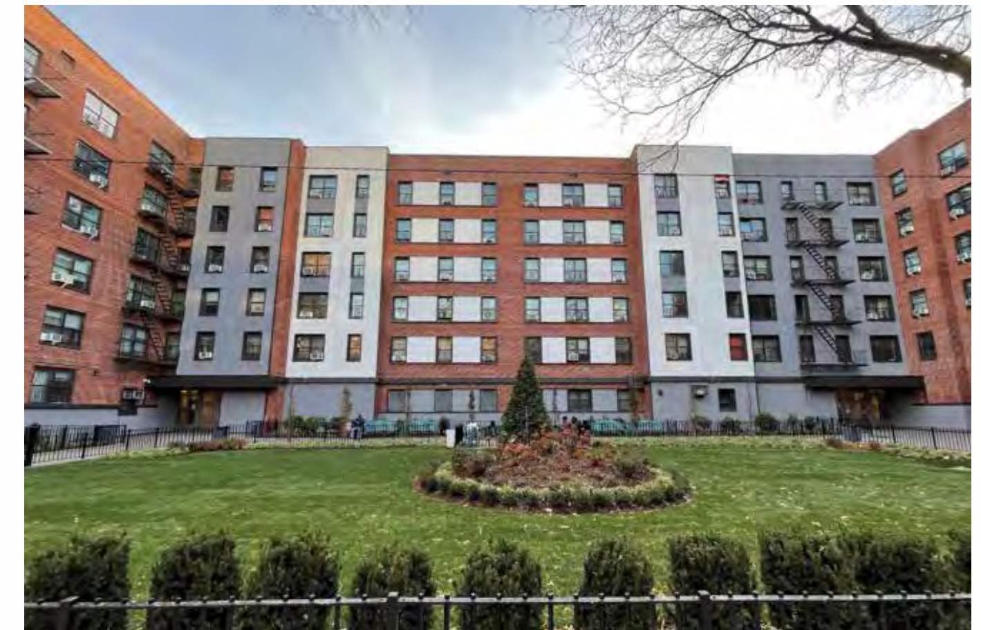
Site improvements at Warren St Houses
