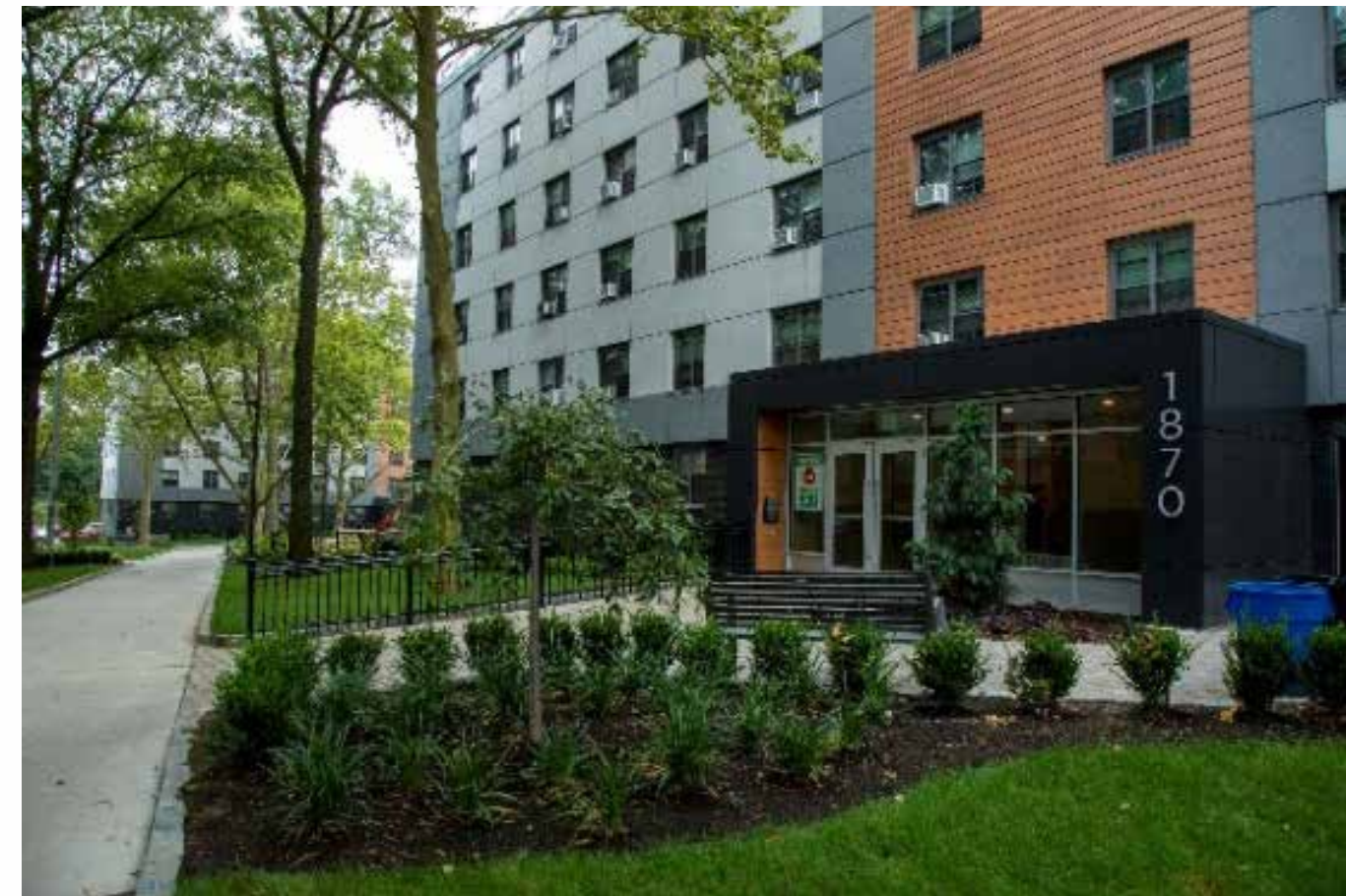
Site improvements at Baychester
