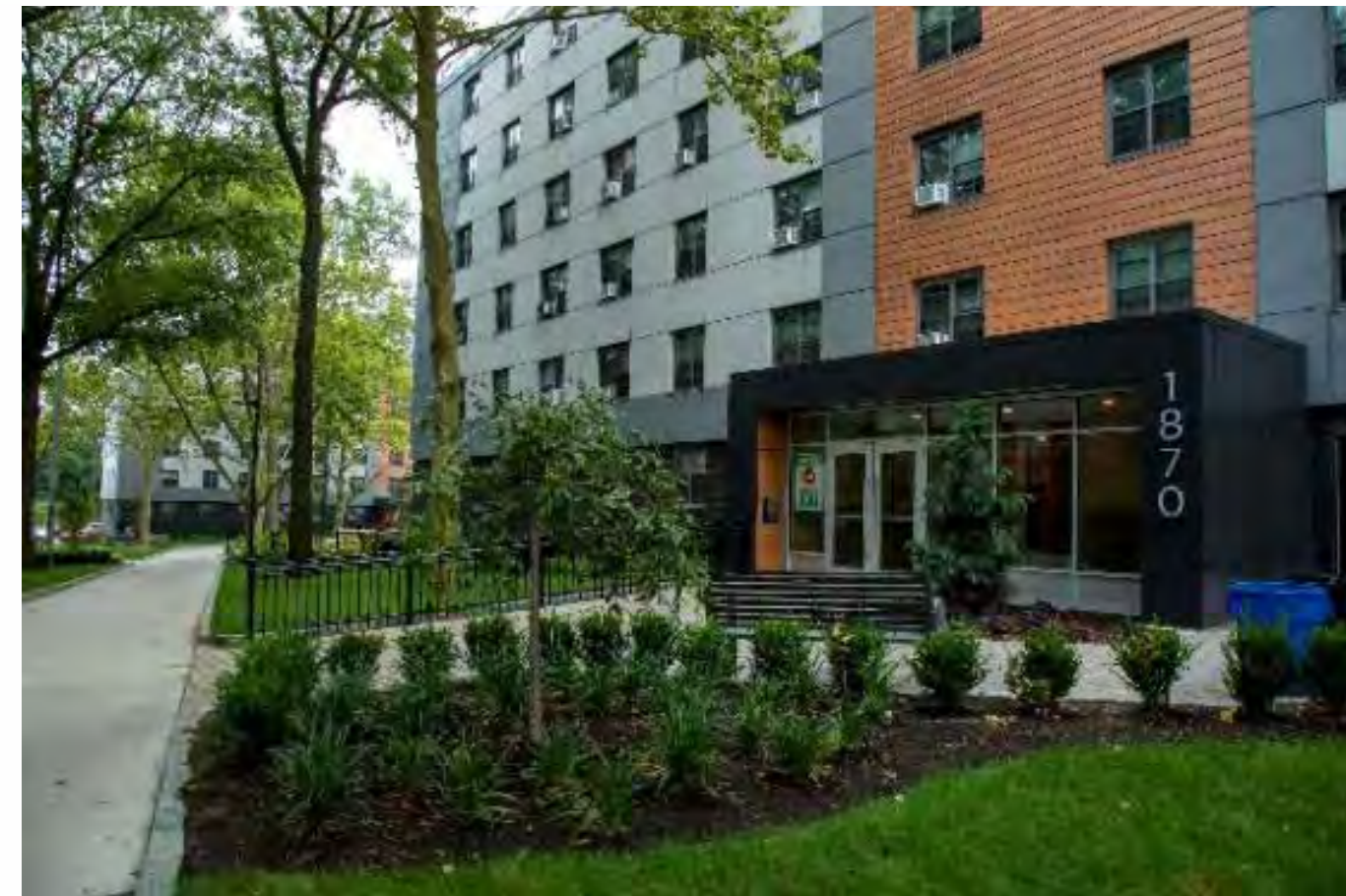
Renovated apartment at Twin Parks West
